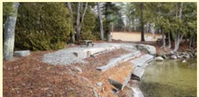
BMP including Erosion Control Mulch, Native Plantings, and Stone were executed at Pleasant Point to impede the flow of sediment into McGrath Pond.
