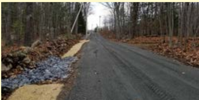
Best Management Practices (BMP) were implemented at Camp Tracy with Bluestone, Rip Rap, Turnouts, and Erosion Control Blankets to help limit runoff.
