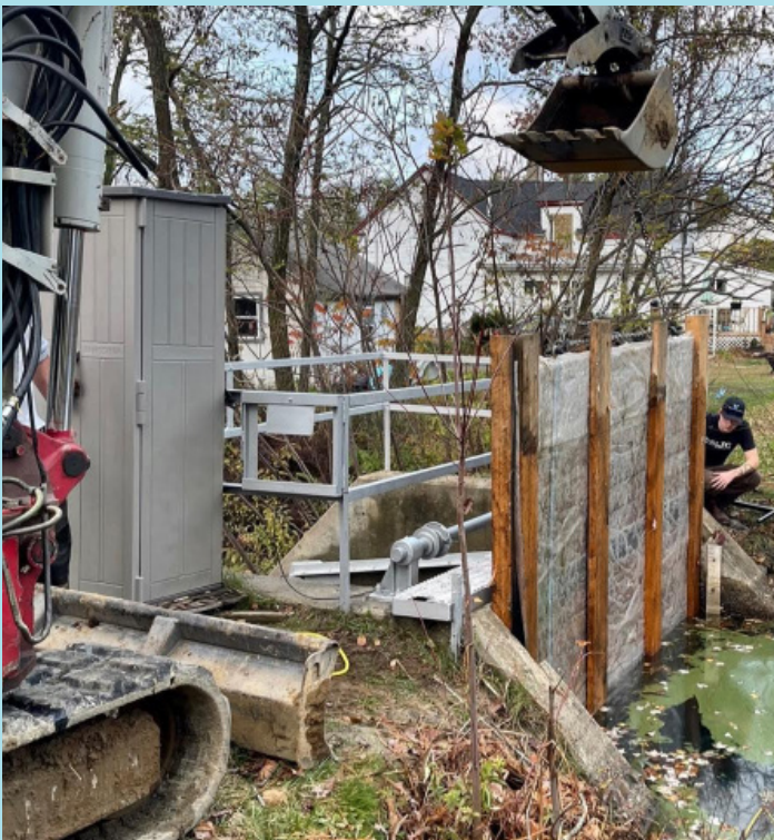
Installation of the temporary coffer dam
