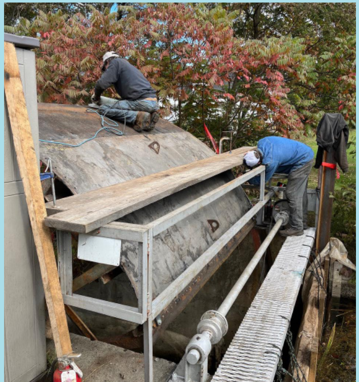
Installation of two 5/16" welded steel plates
