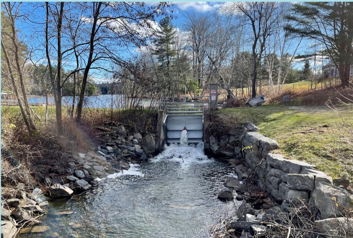
Salmon Lake Dam with the new 1 CFS metered valve
