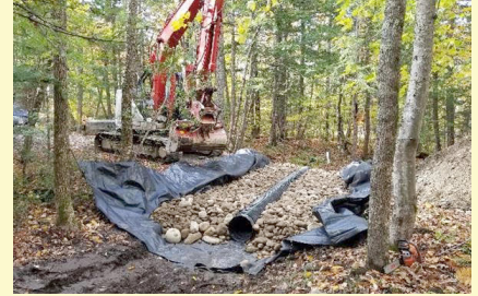
Salmon Lake Culvert with "Rock Sandwich"
